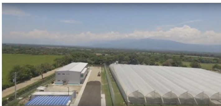
Figure 3: Khiron's Cultivation Facility: Areas for cultivation, mother plants, seeds, cuttings, germination, extraction and QA/QC facilities
